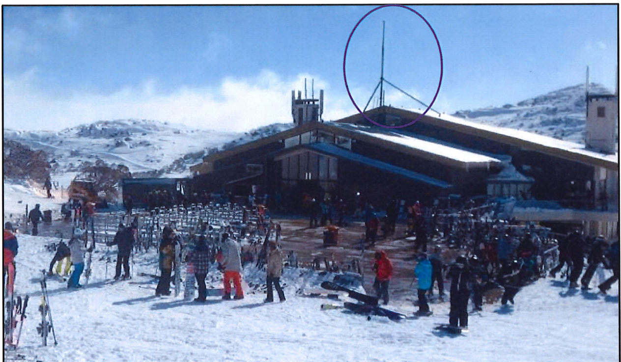
Figure 2: Blue Cow Terminal building and lightning rod
