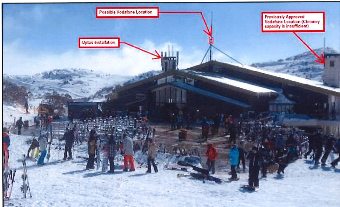
Figure 5: View of building from hardstand courtyard area
