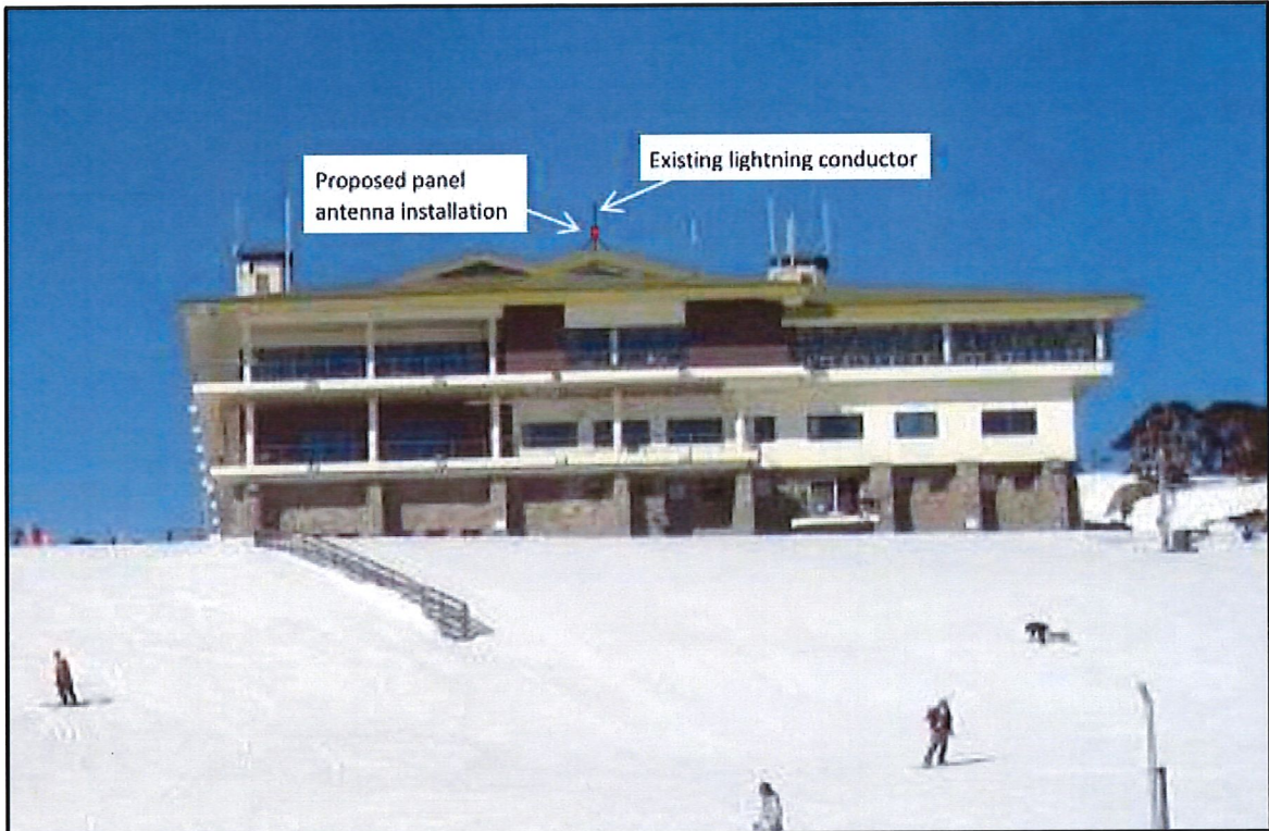
Figure 4: View of building from the ski slope
